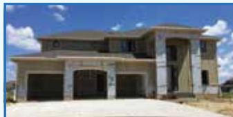
20752 PINE ST Windgate Ranch • $453,450
